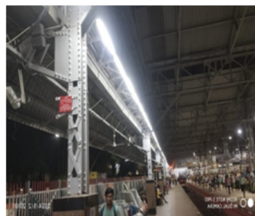
Trunking light arrangement at SDAH
