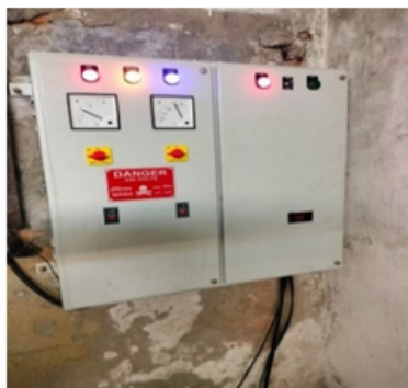
New Pump control panel at JJC
